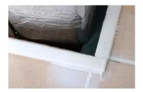
CONIPUR 3335 is applied to the pre-treated surface using a pin squeegee.
