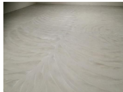
surface with levelling compound
