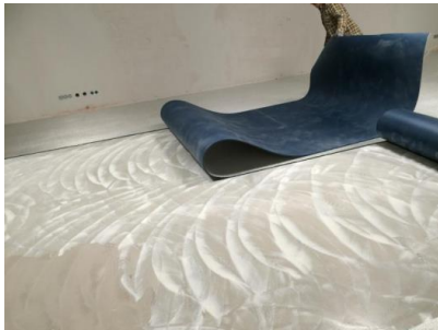
laying of the mat into adhesive
