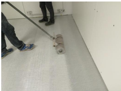
rolling transverse to the length
