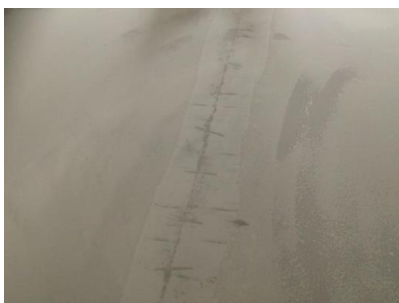
prepared construction joint
